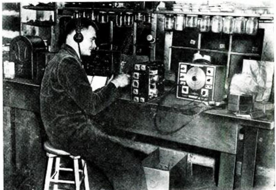
David Crandall, author's co-experimenter, modifies a surplus BC-645 for the citizens band.
